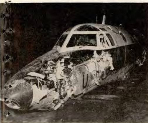
Aircraft sliced through trees, shedding wings, engines and part of tail, but fuselage remained intact. Crew and passengers escaped with only minor injuries.
